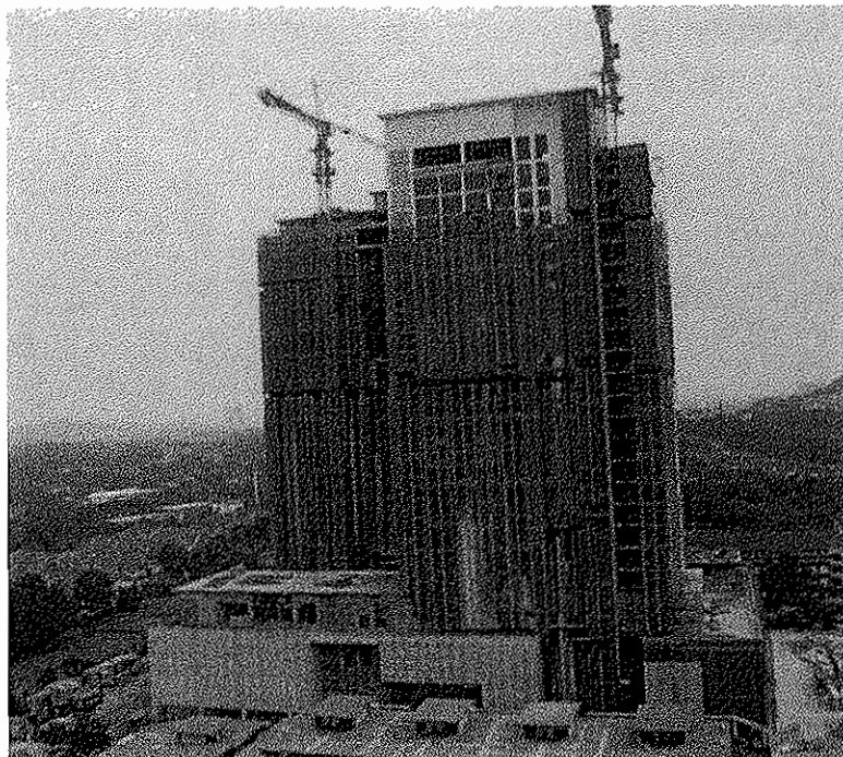
Actual Picture of The Square @ OneCity – Site Progress as at January 2015
